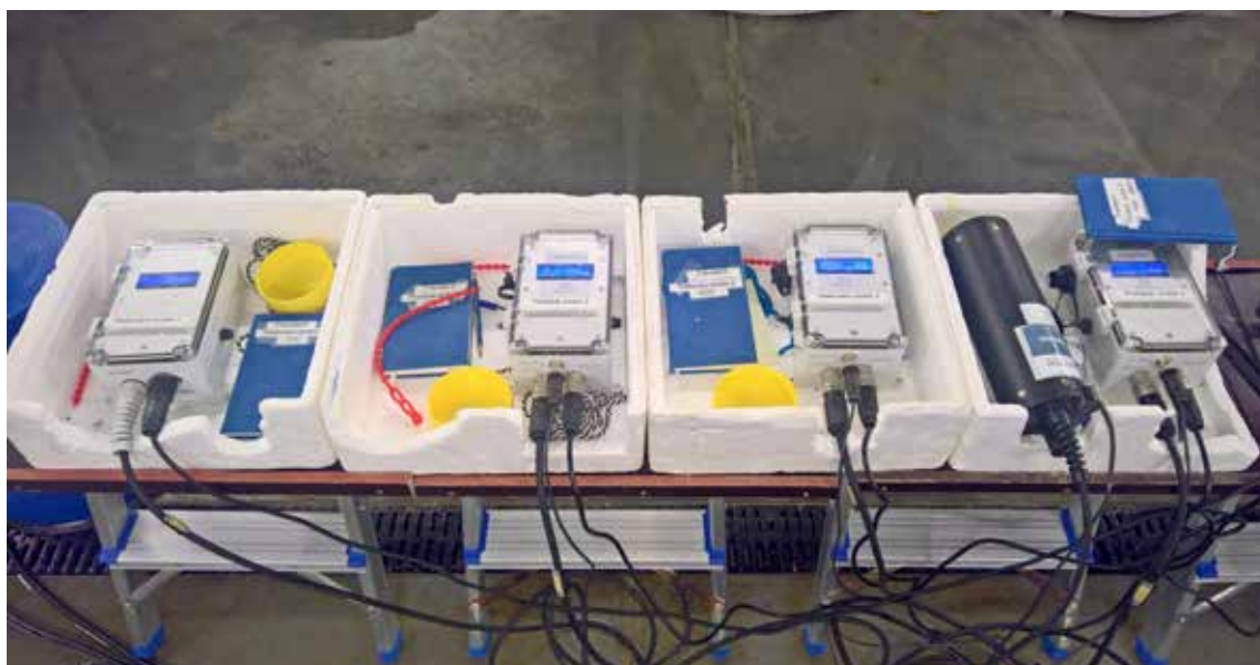
Fig. 4.8. Maintenance and control of sensors is an important and integrative part of rearing fish in closed-containment systems. Photo: Bendik Fyhn Terjesen
